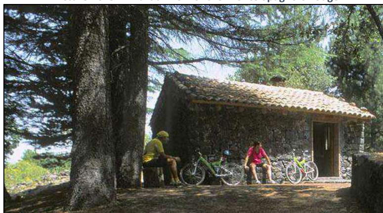
Picture no. 32 – Partial view of the Monte Spagnolo Lodge
