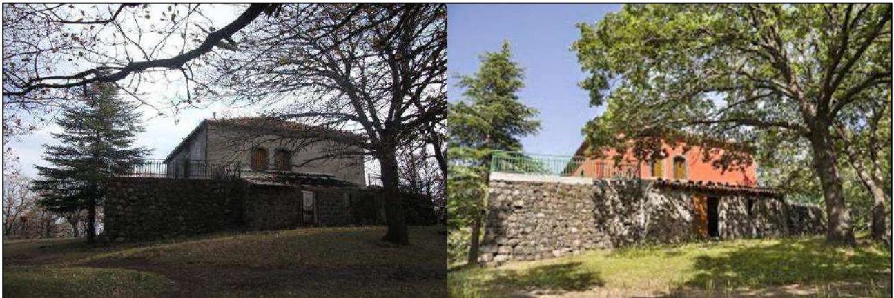
Picture no. 30 - Caserma Pitarrone before and after the restoration process
