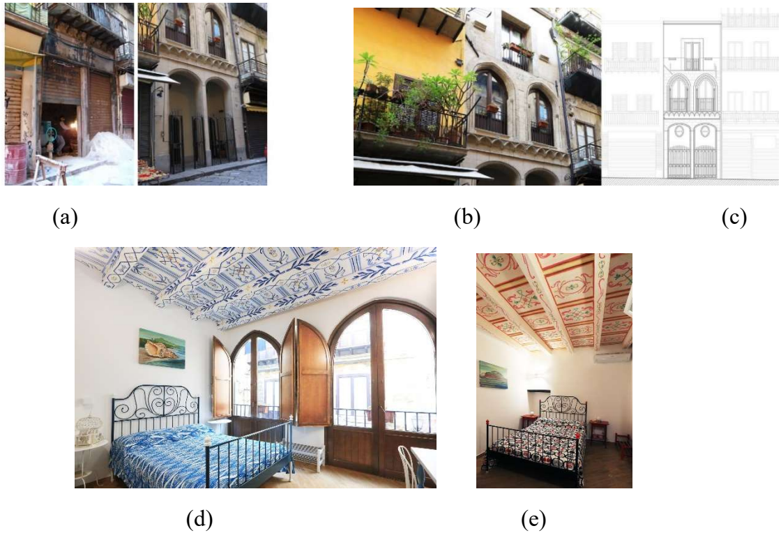
Figure 17: Restoration and renovation of degraded building on in Vucciria – no. 1
