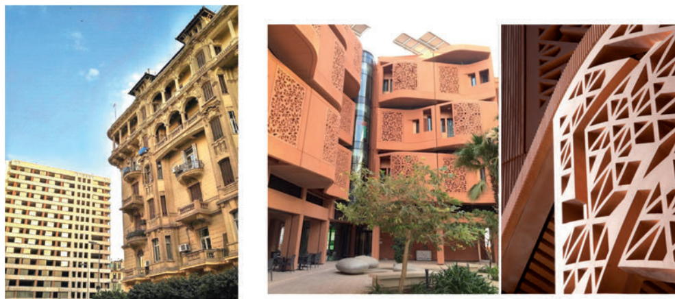
Figure 1. Represents a photograph taken of two different buildings in Cairo, Egypt. It demonstrates the contradiction and the peripheral cursory external façade, thus the loss of architectural identity. Figures 2 and 3. Represent Masdar institute residential facades in Abu Dhabi to demonstrate the preservation of identity through architecture using Islamic geometric patterns and modern technology techniques.
