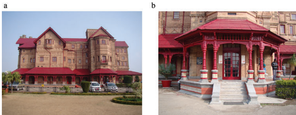
Figure 6. (a) Front façade of Amar Mahal, (b) Use of local material and designs.
