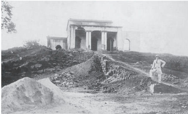
Figure 3(a). The Bashirbagh guest house before intervention.
