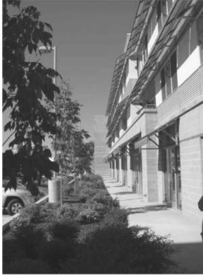
Fig 22: An overview of a building in Artspace Commons project
