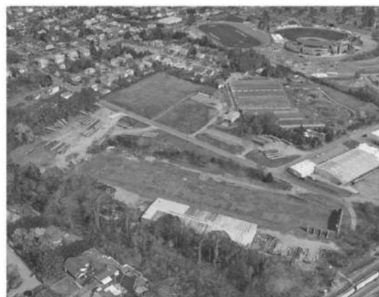
Fig 23: A view of the Allen-Morrison industrial plant ( De Sousa, 2021 )
