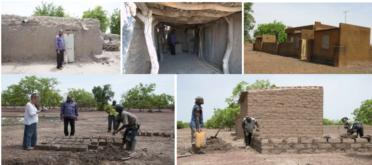
Fig.10: Sanabà. At the top center, exterior and interior views of a dwelling with a raw earth roof, showing the supporting wooden structure, and a dwelling with a corrugated metal sheet roof. In the sequence below, the construction phases of a small house.
