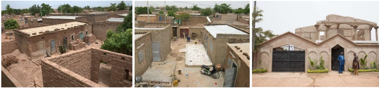
Fig.7: Outskirts of Ouagadougou. On the left, an adobe dwelling; in the center, a house built with concrete blocks; on the right, a single-family villa in reinforced concrete.
