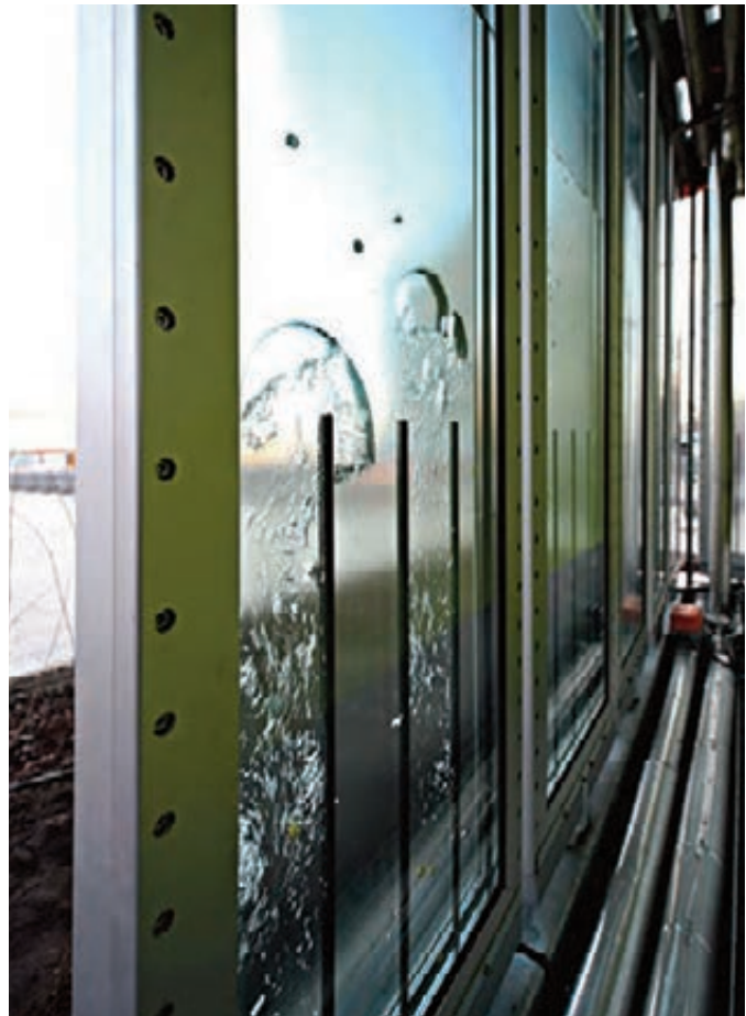
Fig. 1, 2 | Smart Material House BIQ in Hamburg by Splitterwerk Architects and Arup, 2013. The most significant element is the integration, on the south-east and south-west building façades, of flat-screen bioreactors, made up of microalgae (source: syndebio.com/).
