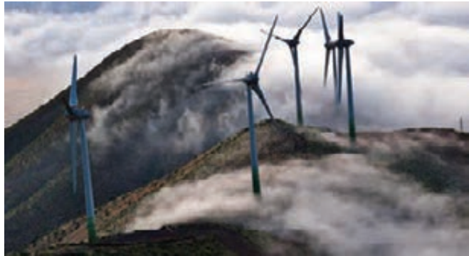
Fig. 30-32 | Wind Turbines and water reservoir, Gorona del Viento, Spain (credits: Renisla, 2014).
