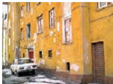
Fig. 1 | Zaharna Fabrika pilot building before renovation (credit: G. Georgiev).
