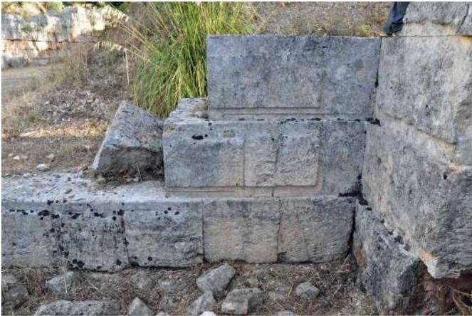
Fig. 36 Segesta, Contrada Mango Sanctuary. Detail of *temenos* wall, with rebates around edges.
