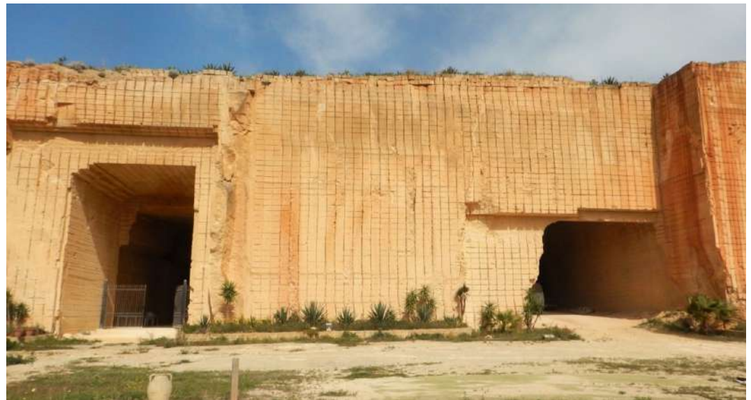
Figure 9. The Foderà Quarry in Marsala, Sicily. View of the entrances of the main tunnels.
