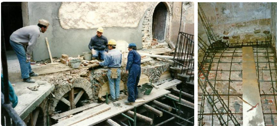
Fig. 5-6: Interventions on the vaults.
