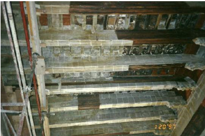
Fig. 13: Intervention to restore a wooden floor.
