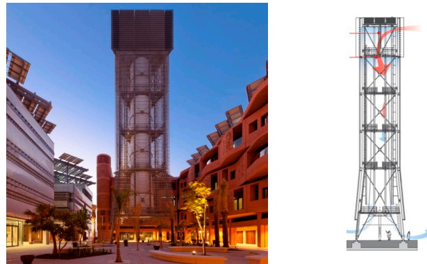
Figure 8. Wind tower in Masdar City, United Arab Emirates, Foster and Partners, Abu Dhabi.
