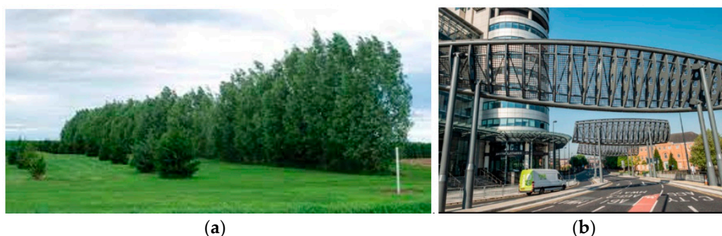
Figure 7. (a) Green barriers at different heights; (b) deflectors made of steel frames covered with perforated aluminum to reduce wind speed, Bridgewater Place, Leeds, England, 2005.
