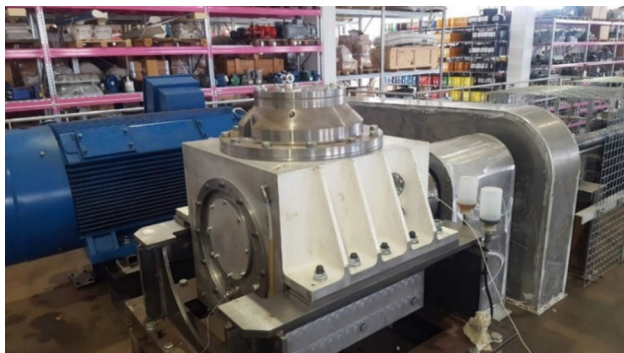
Fig. 7 Connection between the electric motor and the test kinematic chain
