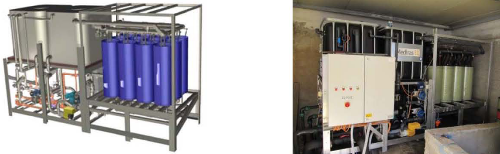
Fig. 2: 3D design and ready installed pilot MD system in Pantelleria
