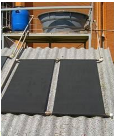
Figure 1: Low cost solar collector system for 100 L
