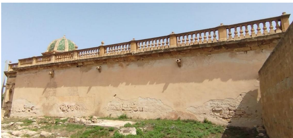
Figure 69. The southern façade of the church from the upper churchyard.
