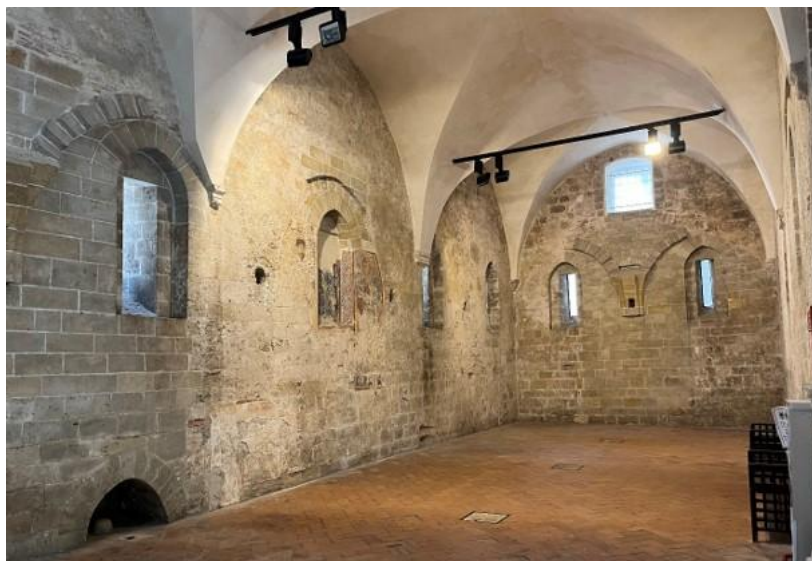
Figure 33. Interior view of the Islamic Hall.
