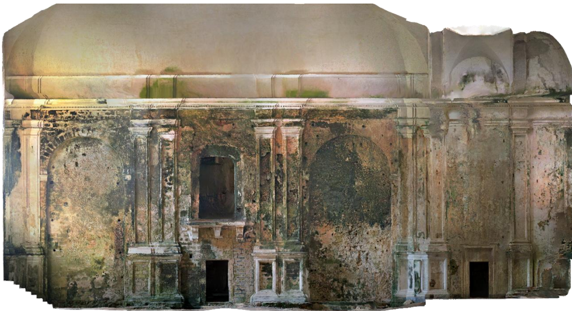
Figure 89. The orthophoto of the internal southern façade.
