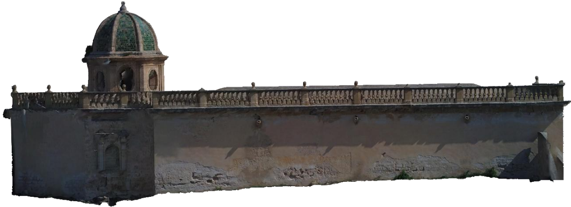
Figure 86. The orthophoto of the external southern façade.
