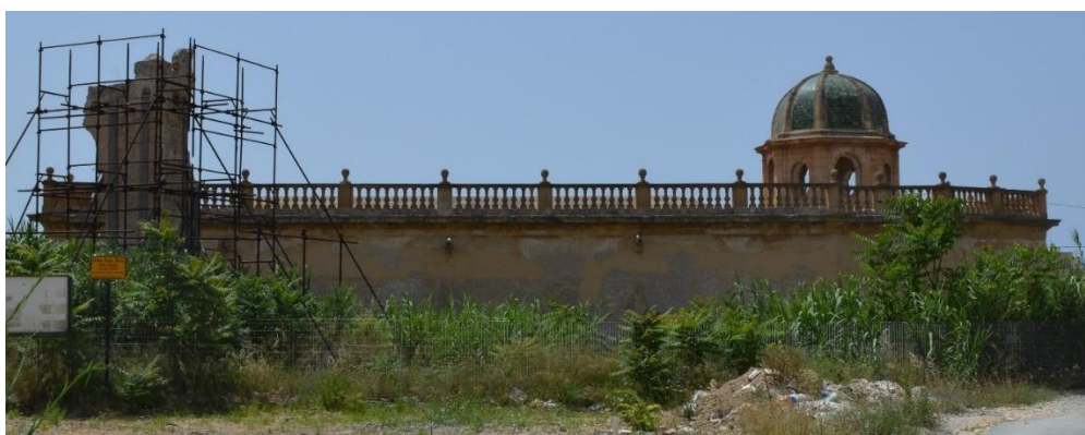
Figure 70. The northern façade of the church from the access street.
