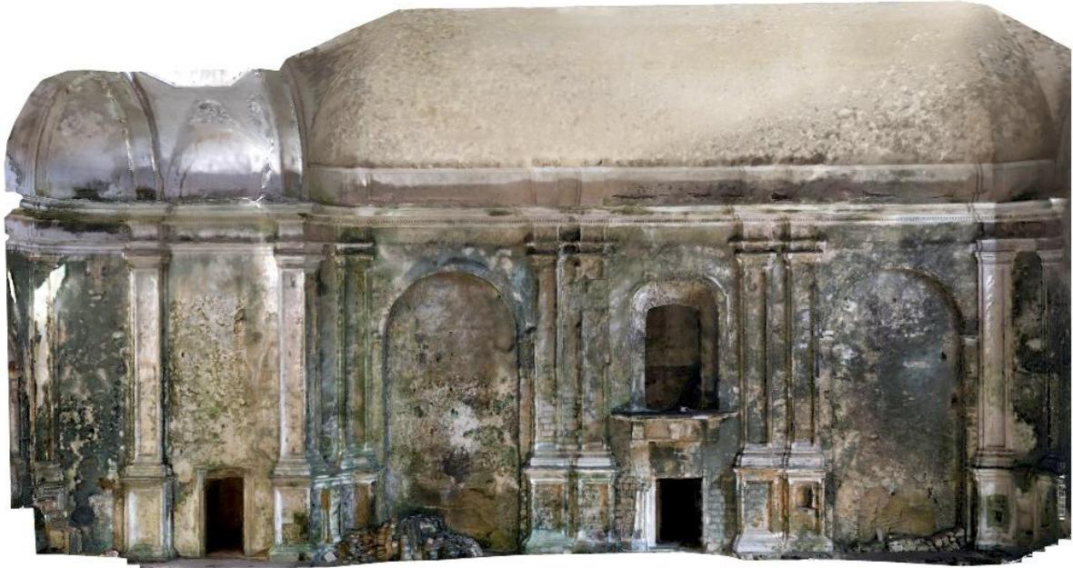
Figure 90. The orthophoto of the internal northern façade.
