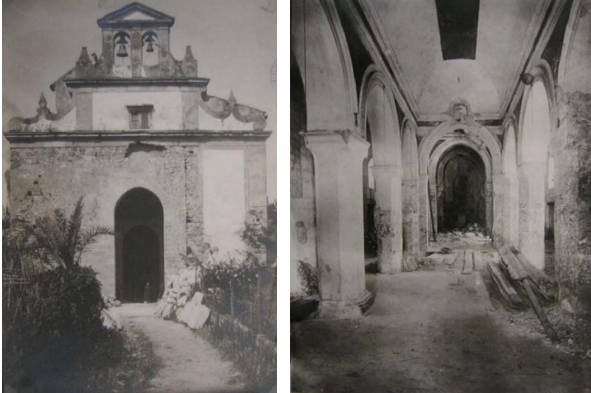
Figure 10. The church before the reinstatement in 1921 (from Genovese, 2010).
