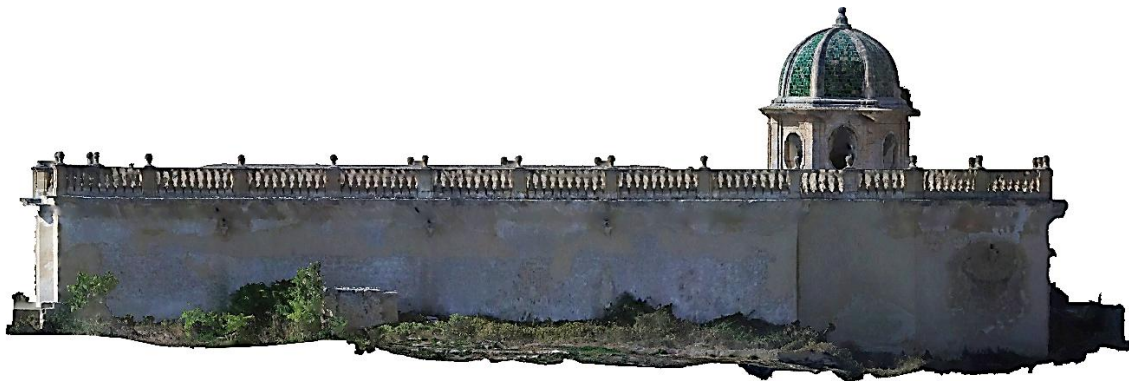
Figure 87. The orthophoto of the external northern façade.
