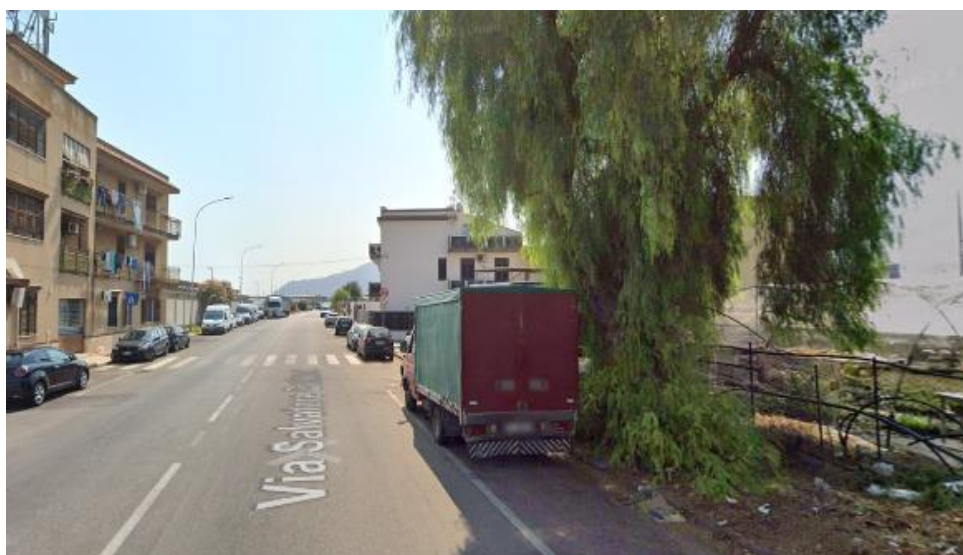
Figure 5–15. Quality of pedestrian infrastructure in the station area; degraded pavement, presence of trees, unsafe crosswalk
