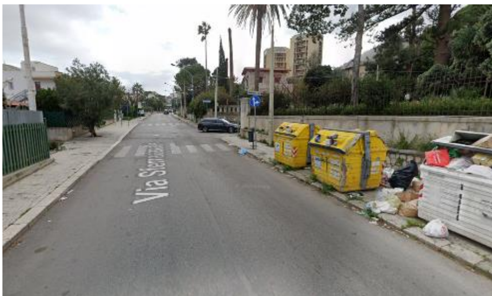
Figure 5–23. Quality of pedestrian infrastructure in the station area; degraded pavement, presence of trash cans, unsafe crosswalk
