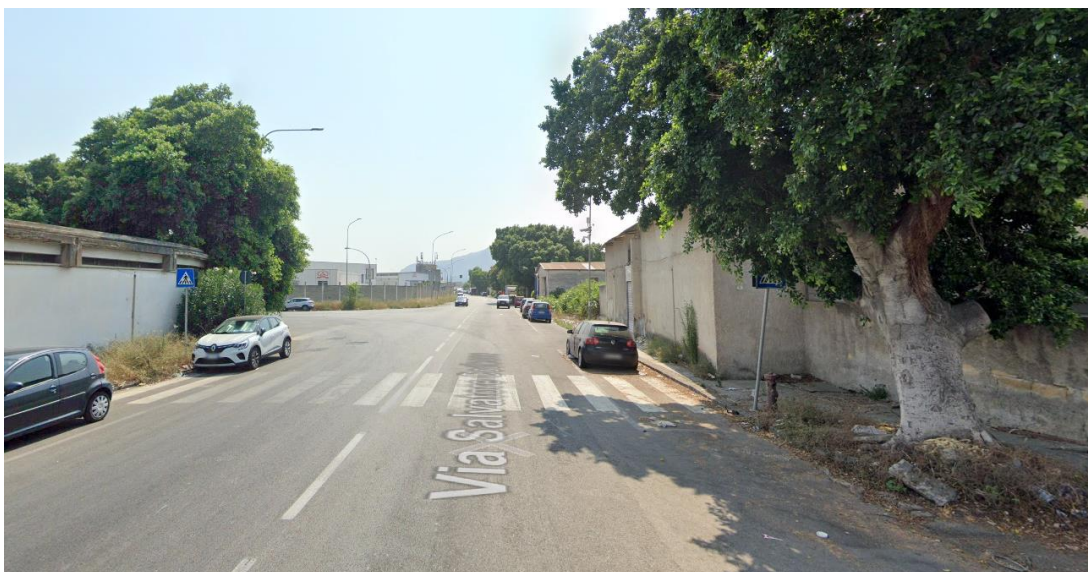
Figure 5–17. Quality of pedestrian infrastructure in the station area; degraded and discontinued pavement, presence of trees, unsafe crosswalk
