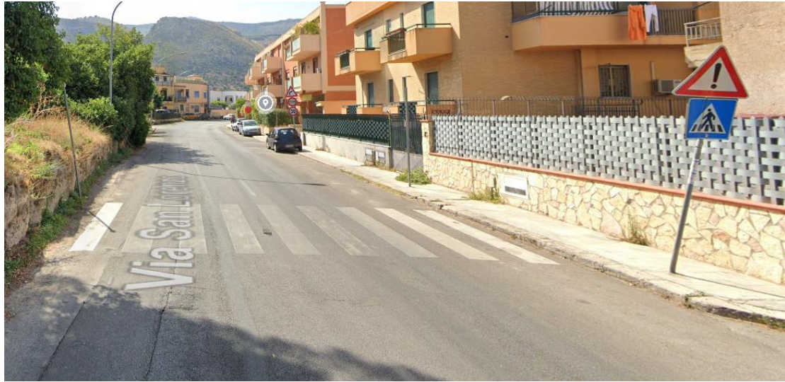
Figure 5–27. Quality of pedestrian infrastructure in the catchment area of the station; no sidewalk present on the left side, presence of trees, and unsafe crosswalk at midblock
