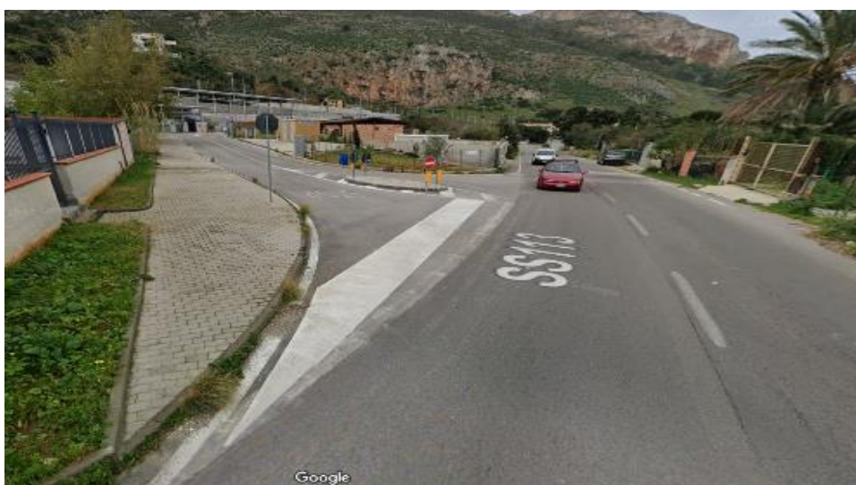
Figure 5–22. Quality of pedestrian infrastructure in front of the station; high-speed roadway, no sidewalk, and crosswalk
