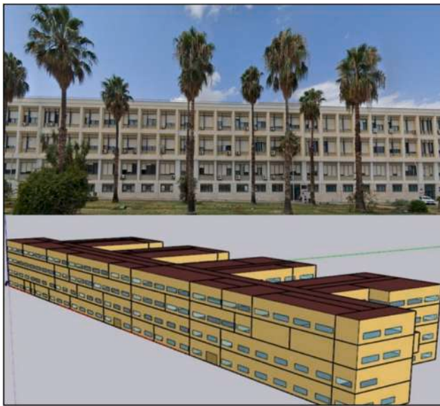
Fig. 3. Building 6 picture and, below, a view of the energy model created with SketchUp 3D Modelling Software (integrated by the Euclid-NREL Energy Plus Plugin).
