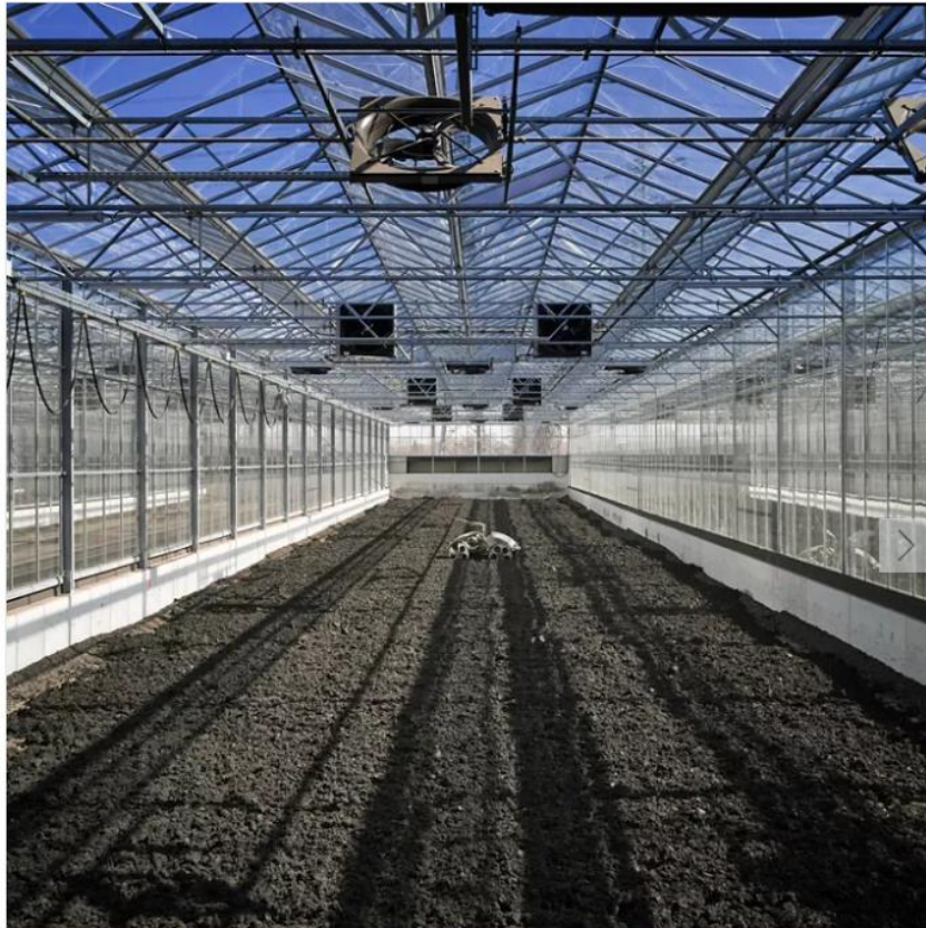
Figure 4.16 - Sludge drying chamber in Bottrop WWTP (adapted from Viega Group, 2021)
