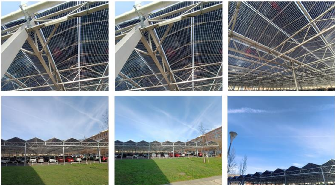
Figure 86 Photovoltaic Installation at parking area: 1.1 MW renewable energy integration.
