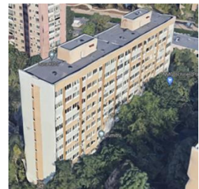
Figure 16 Mid-rise (West-East oriented) residential buildings
