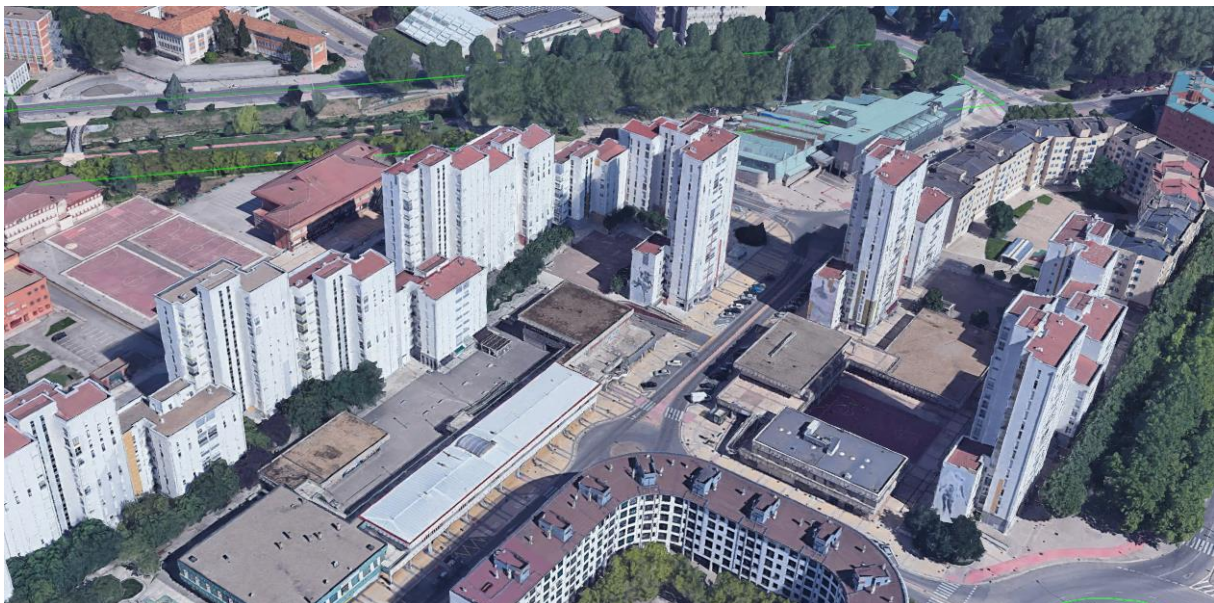
Fig. 20. Sky View of Río Vena District Heating Network Cluster of Buildings [17]
