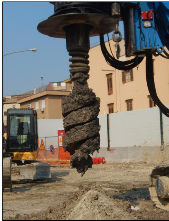
Figure 34: core-destroying drilling.
