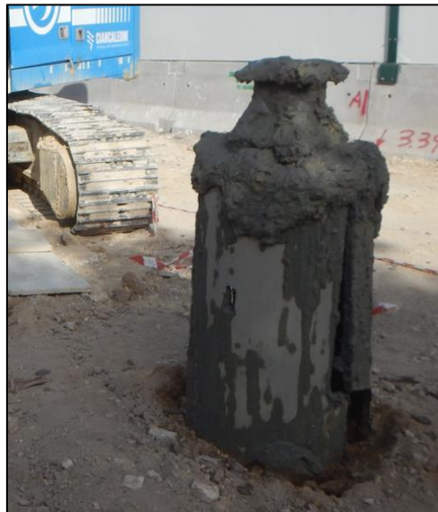
Figure 35: Bucket used to extract soft materials.
