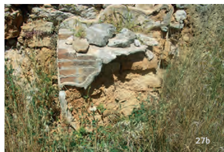
Fig. 25: Solunto. Sanctuary (block 8, unit I); Hellenistic-Roman period. Adobe wall patched-up with cement in the 1950s. Remarks by M. Schiera 2006.
