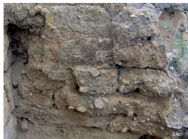
Figs. 24a-c: Solunto. Block 12 –unit V. Residential building; Hellenistic-Roman period. Details of the part in raw earth, with traces of cement covering of the crest (ca 1955) (photo by M. L. G. 2006).
