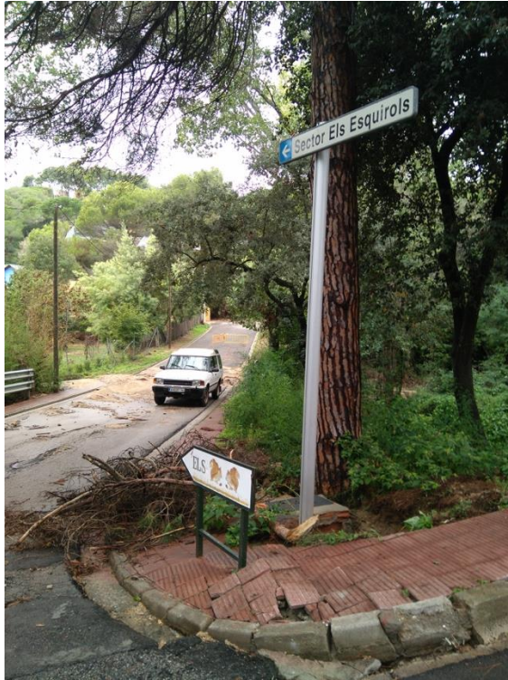
Figure 8 - Damages to the pavement caused by floods in Vilassar de Dalt (Source: FLOODUP).
