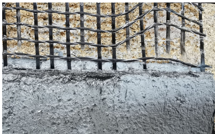
Figure 3.49: Observed failure mode E1 for specimens of group BC_DSB2.
