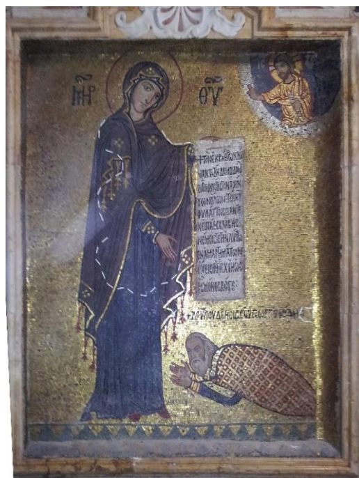
Figure 3. Palermo, St. Mary of the Admiral, Dedication mosaic panel: George of Antioch prostrate at the feet of the Virgin Mary. The hatched lines indicate the areas affected by the risk of detachment of the tesserae, as previously indicated by the restorers.
