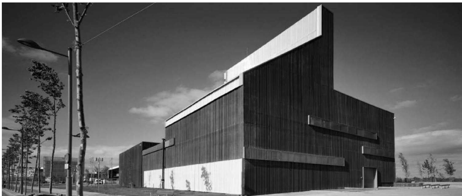
1 Iñaky Alday, District Heating & Cooling, Water Park, Zaragoza, 2008
