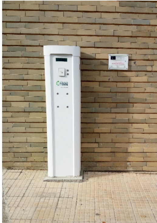
Figure 12.5. An energy charging station fed by a PV plant.
