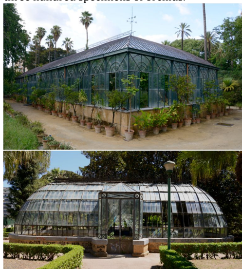
Fig. 9 - Above, the Botanical Garden greenhouse; below the greenhouse of the English Garden in the current conditions (Photo C. Bustinto).
