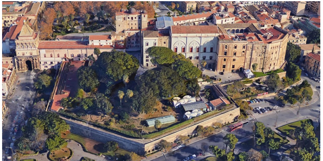
Fig. 1 - Hanging garden on the bulwark of San Pietro
