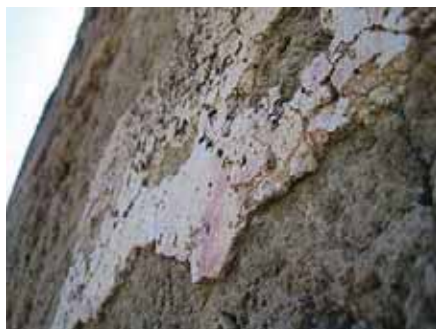
Fig. 06 : Santa Maria in Campogrosso, detail of the plaster in the inner part of the masonry of the central apse
