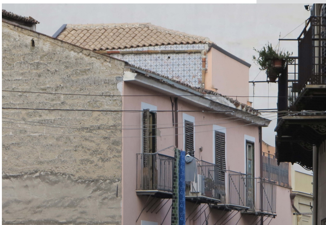
Figure 4. Building in discesa dei Giudici. The additional storey at top of the construction is located behind the building façade. The transverse wall, oriented to the West, is covered by enamelled tiles.
