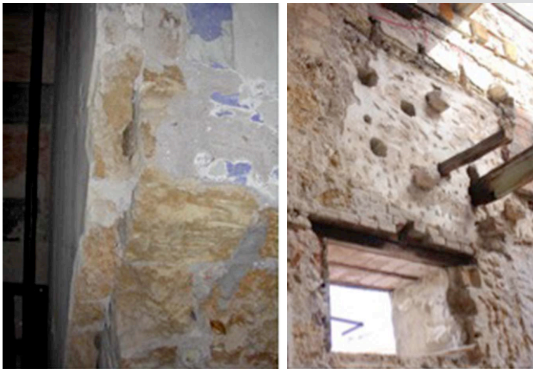
Figure 3. Additional calcarenite (left) and brick (right) masonry, intended to increase the wall thickness. On the right, connection blocks are visible.
