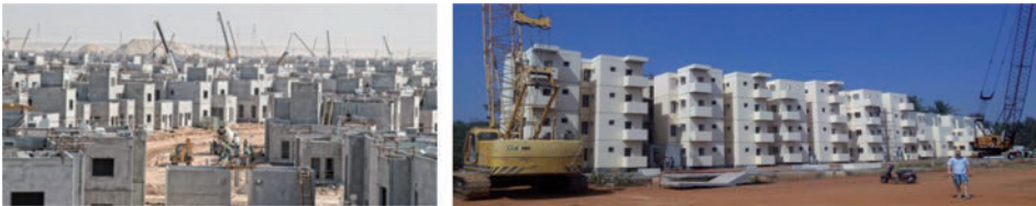
Figure 14. On left & right, illustrate housing compounds constructed with precast concrete. (Zuhairi bin Abdel Hamid).
