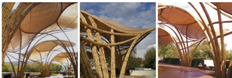
Figure 6. Pictures for the pavilion constructed in Zaragoza, Spain in 2008.
