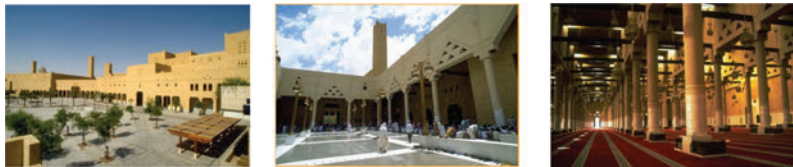
Figure 4. Great mosque. The source: http://www.akdn.org/ru/architecture/project/great-mosque .
