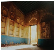
Figure 41. General view of the reception room in the Hussein Rifai house.
