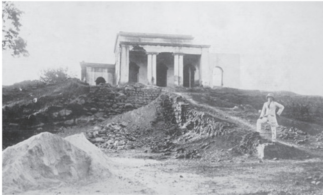
Figure 3(a). The Bashirbagh guest house before intervention.
