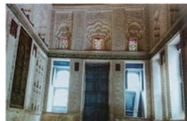
Figure 30. Stucco decorations, calligraphic streaks, and stucco sunshades with stained glass in the sitting hall of the Ahmed Munawar Rifai house (AD 1922).
