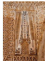
Figure 39. Stucco details of one of the side entrances of the Hussein Rifai house.
