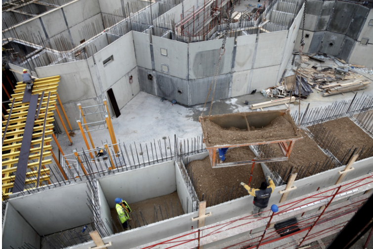
Figure 2.1: Accelerator building construction applying Forster Sandwich Construction technology.
